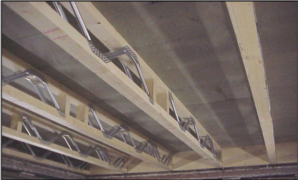
Photograph 6. View from below, before FireLine boards and noggings were attached.
