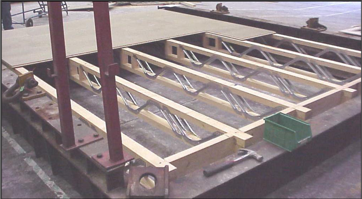
Photograph 5. Ecojoists in position with chipboard walking surface being fixed into position.
