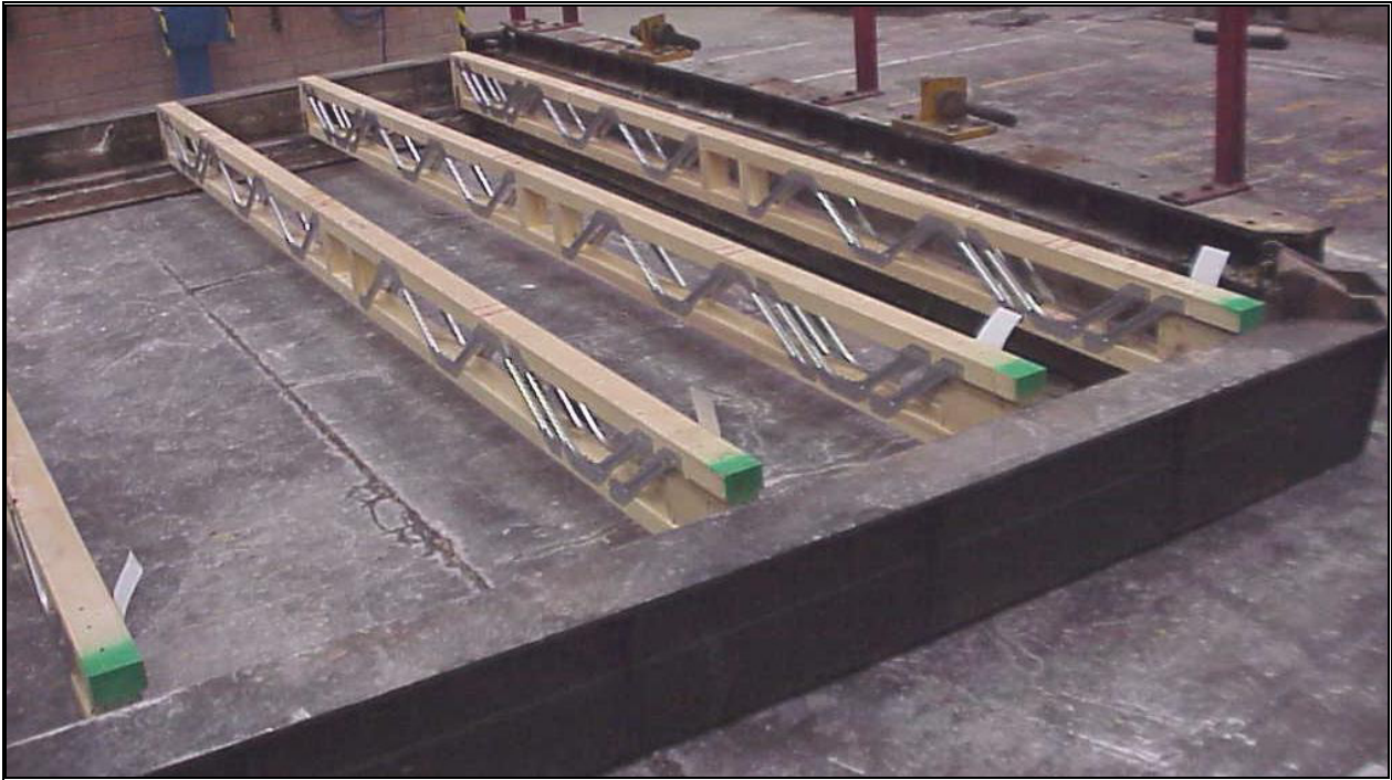
Photograph 4. Ecojoists positioned across the 4m length of the test frame.
