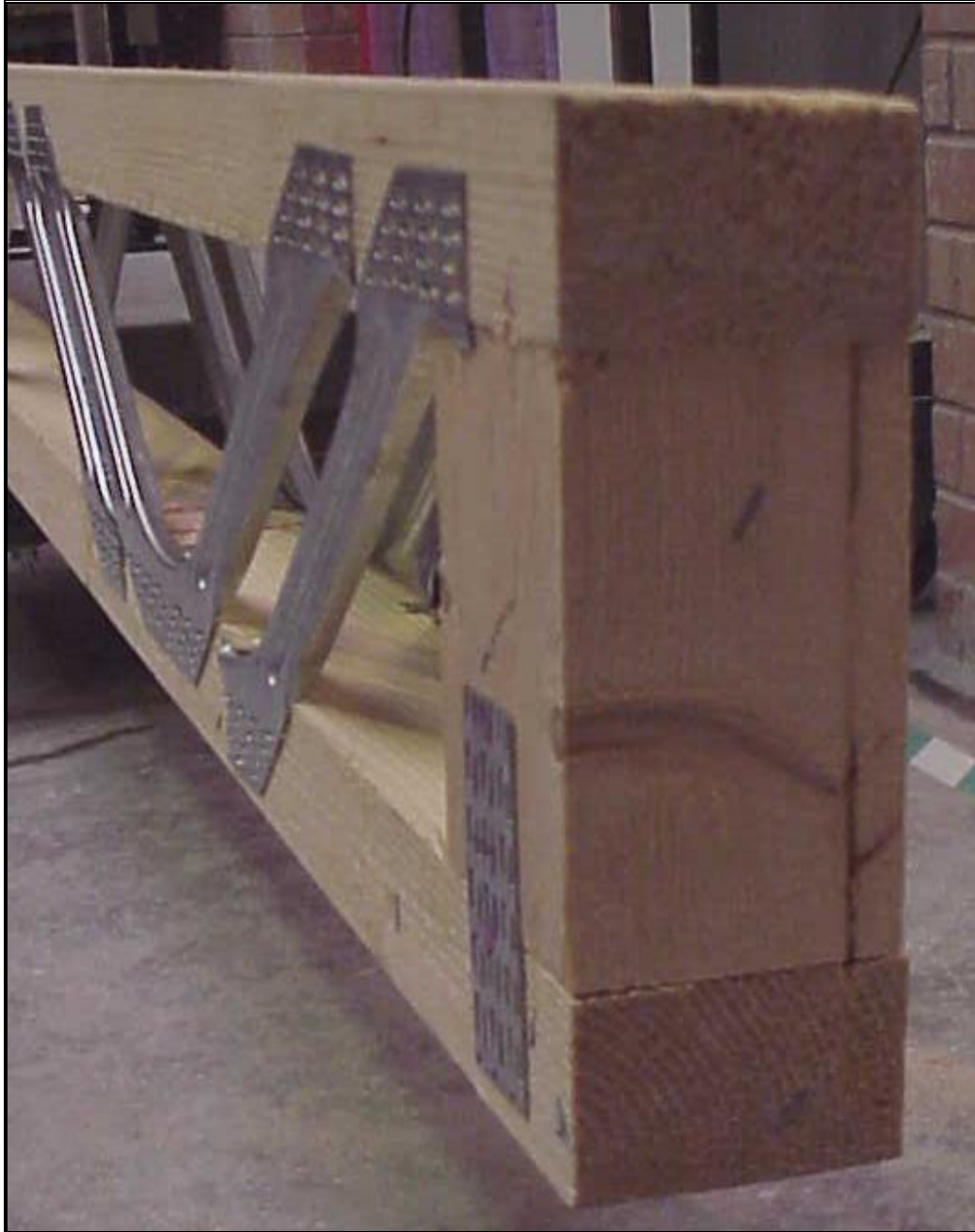
Photograph 3. End view of Ecojoist.
