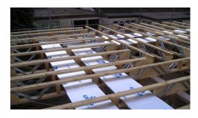
Using Ecojoist as the bottom chord increases the overall floor zone depth due to the requirement to rotate the top and bottom chords of the joist to match that of the remaining attic timbers. With the webs taken into account, the overall depth of the bottom chord increases from 222mm to 353mm.
